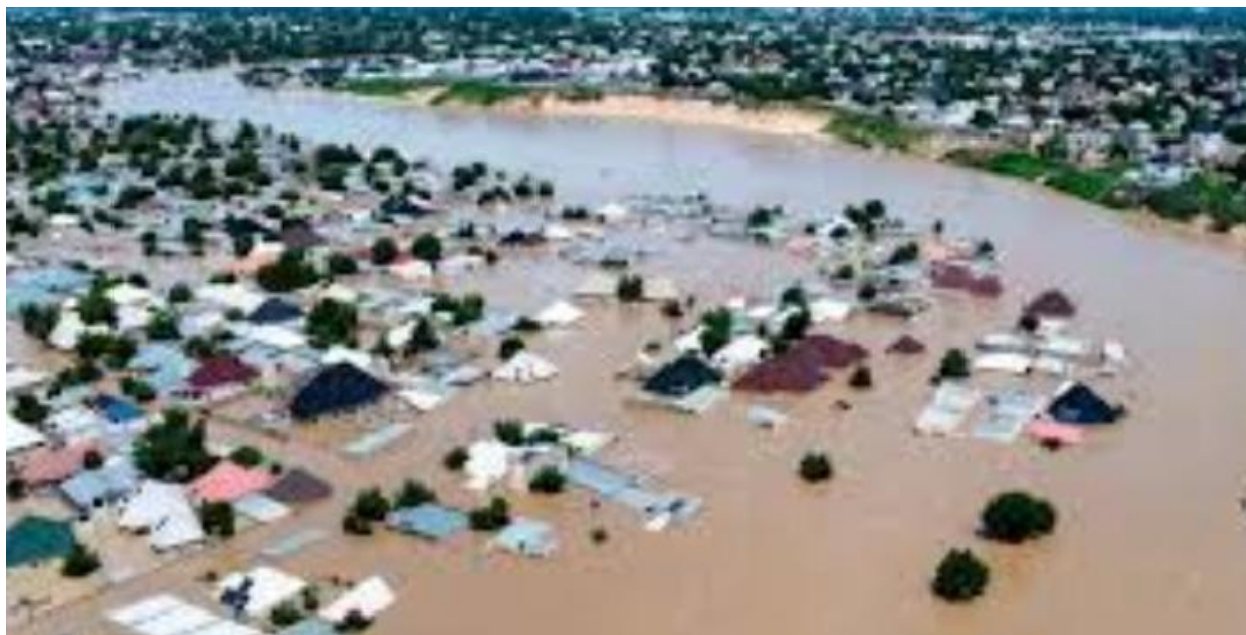
Photo 1: Human settlements affected by floods caused by heavy rain
